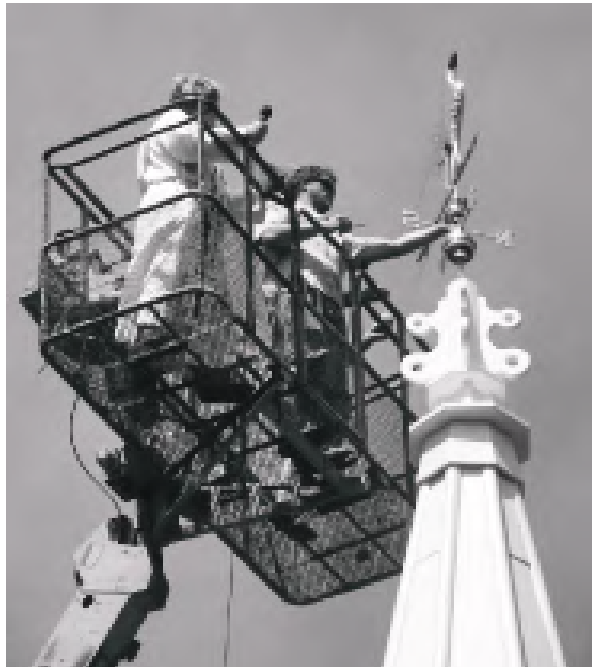
On Sunday, June 11th - Mother Mary Staley from St. Paul's Episcopal Church rode a lift to the top of St. Paul's newly renovated steeple to oversee the placement of a new rooster weathervane. With her in the lift were Rob LaPlante and Billy Borgland who did the work on the steeple.
