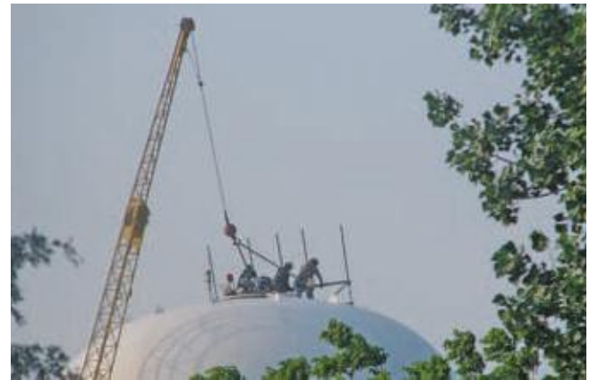
Workers in June putting a new cellphone antenna on top of the Put-in-Bay watertower. Look up. Just look up, and you will see it.
