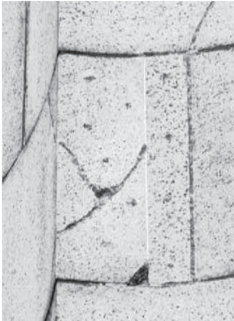
ABOVE: This close-up photo shows an example of the repairs workers were making on the Monument this spring. This piece of granite block was cracked and in danger of falling. From their scaffolds, workers repaired numerous areas of the fluting by pinning and "gluing" the pieces so they would be stabilized and not fall. The black dots on this piece of granite are where the workers put in pins. You can see also see the severe cracks in this particular piece of granite.
