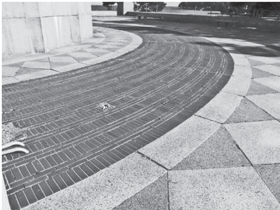
LEFT: This photo shows the stone and brick on the upper plaza at the base of the Monument. Bricks in the design are missing, plus the granite stone pieces have heaved and pose a trip hazard. It will take several million dollars to take all this up, remove the concrete roof over the basement it sits on, pour a new waterproof roof and then replace the brick and granite paver stones. Each year Congress budgets money for the National Parks, but it is never enough to fix everything, so parks compete for repair dollars. Superintendent Blanca Stransky hopes the project will get funding as soon as possible.
