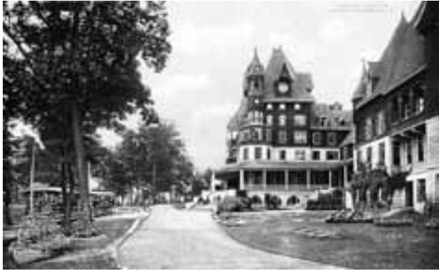
Front of the Hotel Victory with trolley car.
