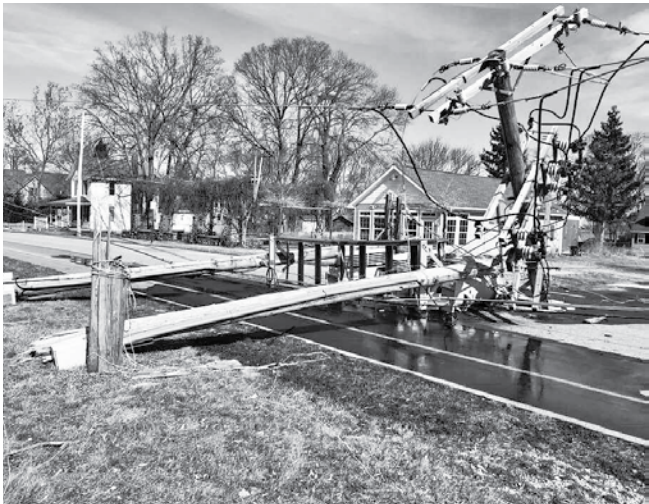
ABOVE: Terry Jenkins from Ohio Edison took this photo of the downed poles across the street from DJ Parker's ice cream shop. The poles came down at the end of February in the worst storm of the winter. It took several days to clean everything up and to reopen the road. In all our years at Put-in-Bay, we have never seen downed poles from the wind like this.
