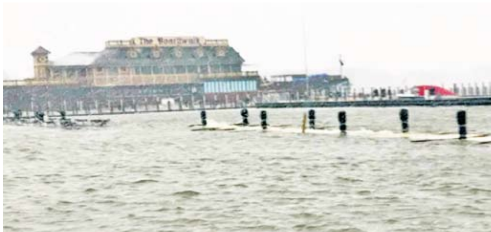
ABOVE: Water was flowing freely over the DeRivera and Village docks during a storm in March which had northeast winds topping 40 miles per hour from time to time. You can see the Boardwalk in the distance. The dock where the Sonny S ferry to Middle Bass ties and where the gas pumps are located was awash with frigid lake water.
