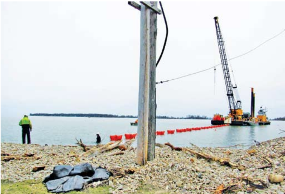
ABOVE: This photo shows the barge being used to lay a new underwater electric line to North Bass from Middle Bass in April. The barge is seen here off the North Bass dock. The line from Middle Bass Island goes into the water at the end of Fox Rd. The new line was installed to replace the old one which dates back to 1956. Interestingly, there are still those who remember when the first electric line was put under the lake to the island. The cost of the new line is $1.2 million, or to put it in other terms, that's about $100,000 per North Bass resident.
