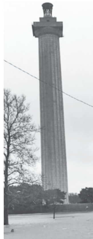
RIGHT: That big storm in mid-April really surprised us. When we looked at our photos, we noticed the Monument appeared to be leaning in the wind.
