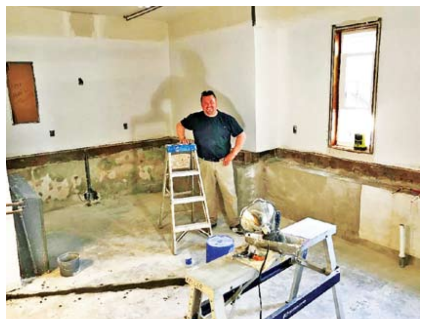
ABOVE: This is how the kitchen looked at the end of April. In the picture is Dave Zilch from Roger Miller Builder, Inc. who is managing the entire Project
