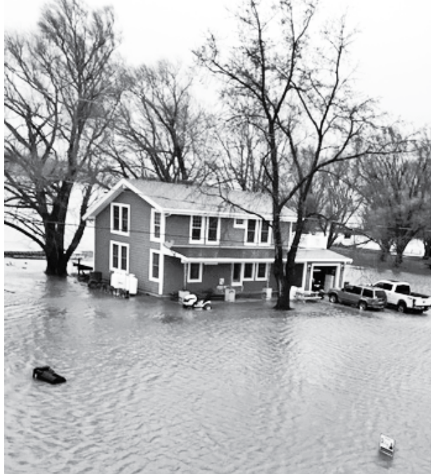
ABOVE: This home at Burgundy Bay was surrounded by the rising water of the northeast storm that hit the islands in mid-April. Years ago when Burgundy Bay was first developed, there was a swimming pool beside the clubhouse building a short distance from this home. When the storm was over, the pool was filled with beach stone. That pool had to be abandoned and moved.
