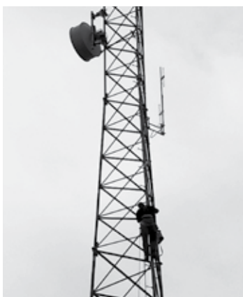
Mi2 relocates radio repeater.
